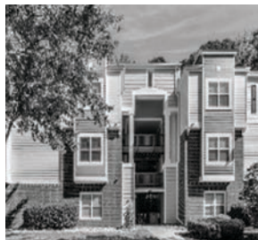
USV I – Hamilton Ridge Multifamily
